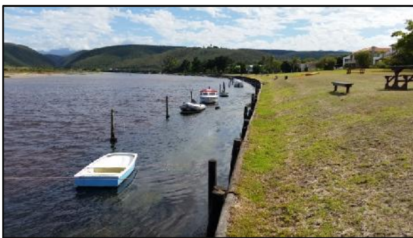
Creosote timber retaining wall and mooring poles that currently exist on Silverstreams Estate. This is not ideal as it results in owners trampling the intertidal zone at low tide to reach their boats.
