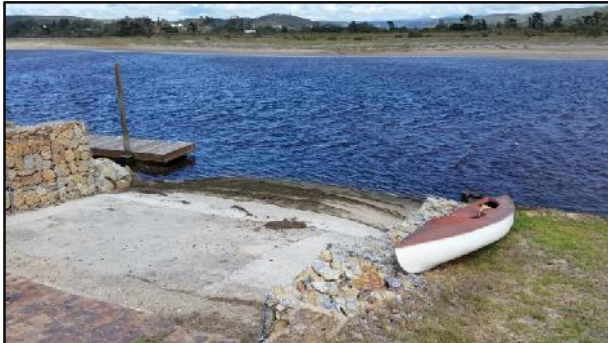
Existing slipway and recently upgraded retaining structure and floating jetty on Blue Waters Estate (adjacent property).
