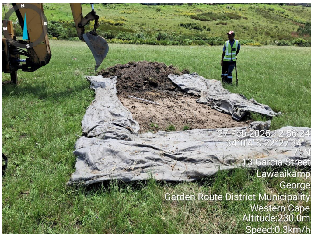
Figure 1 Example of stockpiling topsoil
