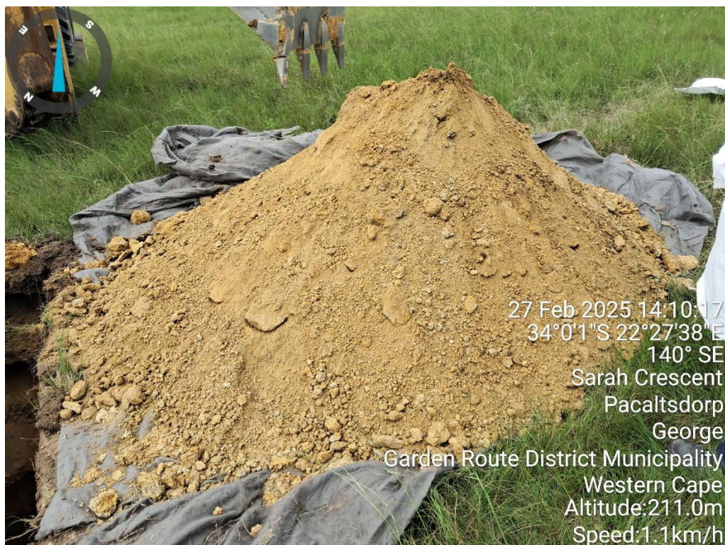
Figure 2 Example of stockpiling in-situ material
