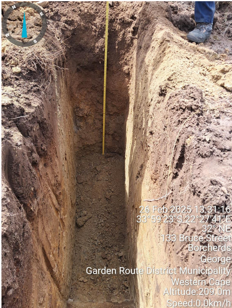
Figure 3 Example of typical test pit
