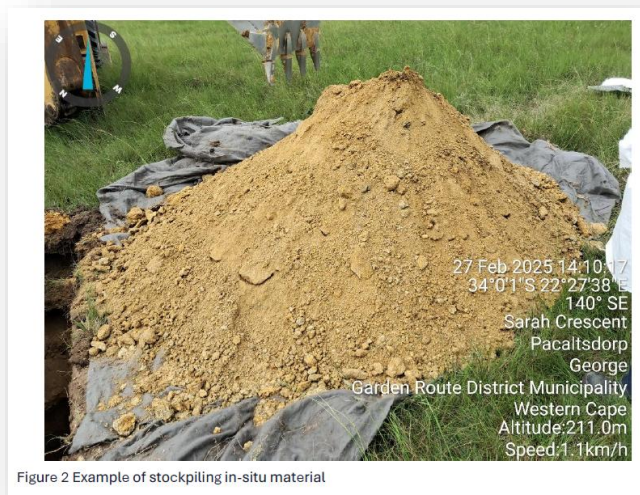
Figure 2 Example of stockpiling in-situ material
