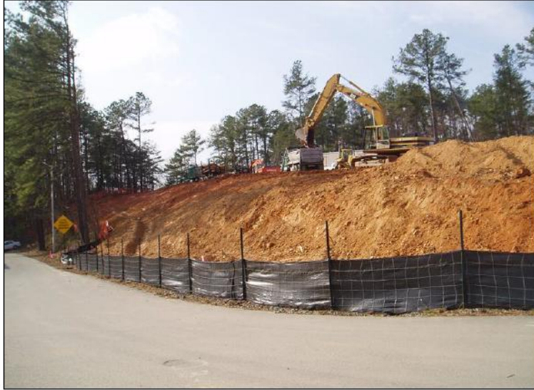
Figure 23. Example of silt fence attached to perimeter fence of a construction area.
