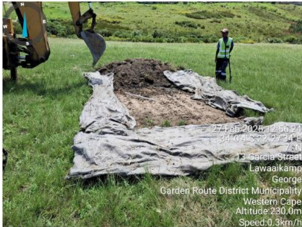
Figure 1 Example of stockpiling topsoil
