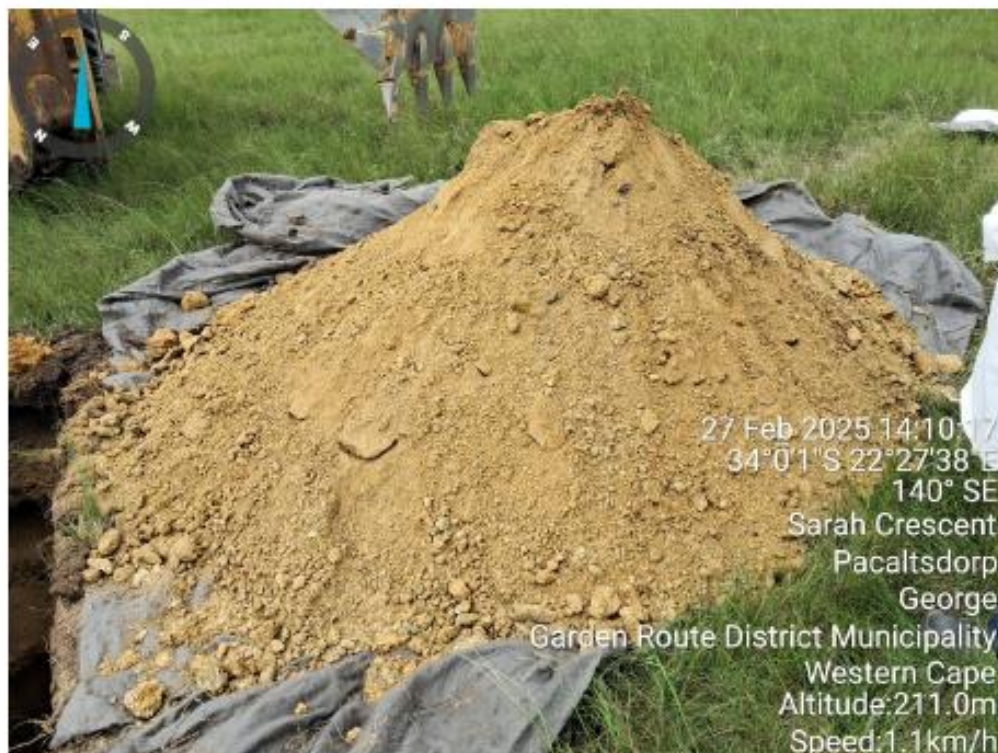
Figure 2 Example of stockpiling in-situ material
