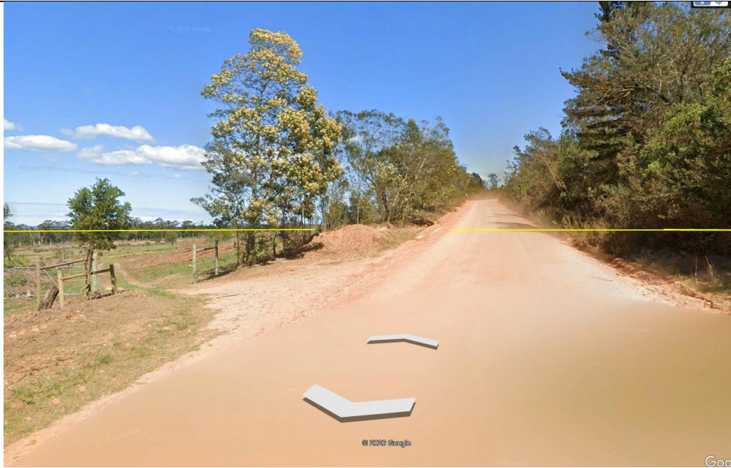
Figure 22 View of the existing farm gate off the DR340 – note the elevation difference and the screening vegetation along the road in the road reserve - (note alien clearing still needs to be undertaken by District Roads in the road reserve).
