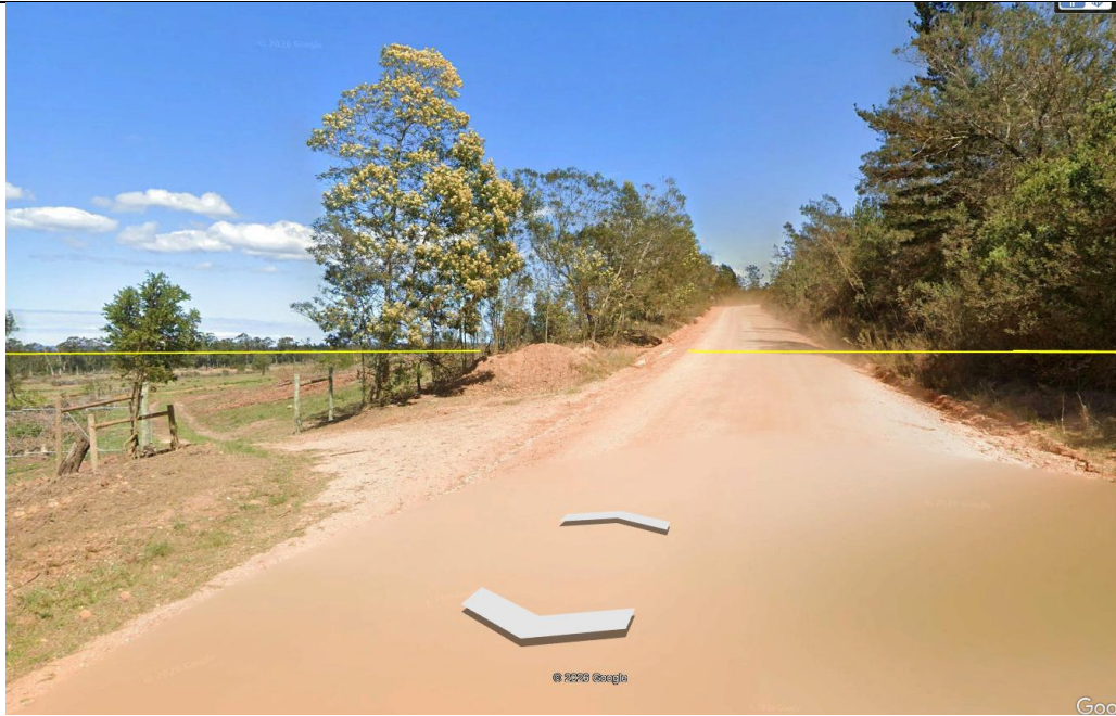
Figure 36 View of the existing farm gate off the DR340 – note the elevation difference and the screening vegetation along the road in the road reserve - (note alien clearing still needs to be undertaken by District Roads in the road reserve).
