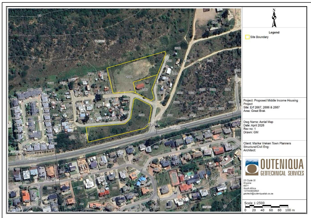
Figure 2: Aerial photo of site area
