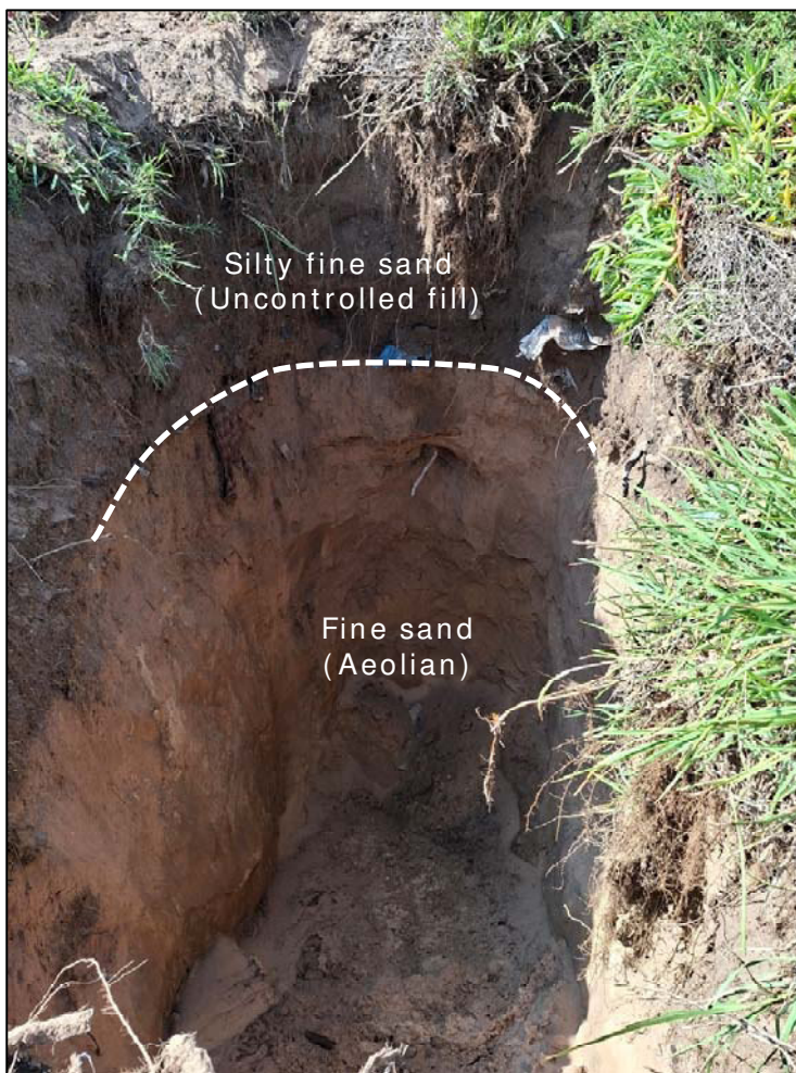
Figure 16: Uncontrolled fill underlain by insitu sand
