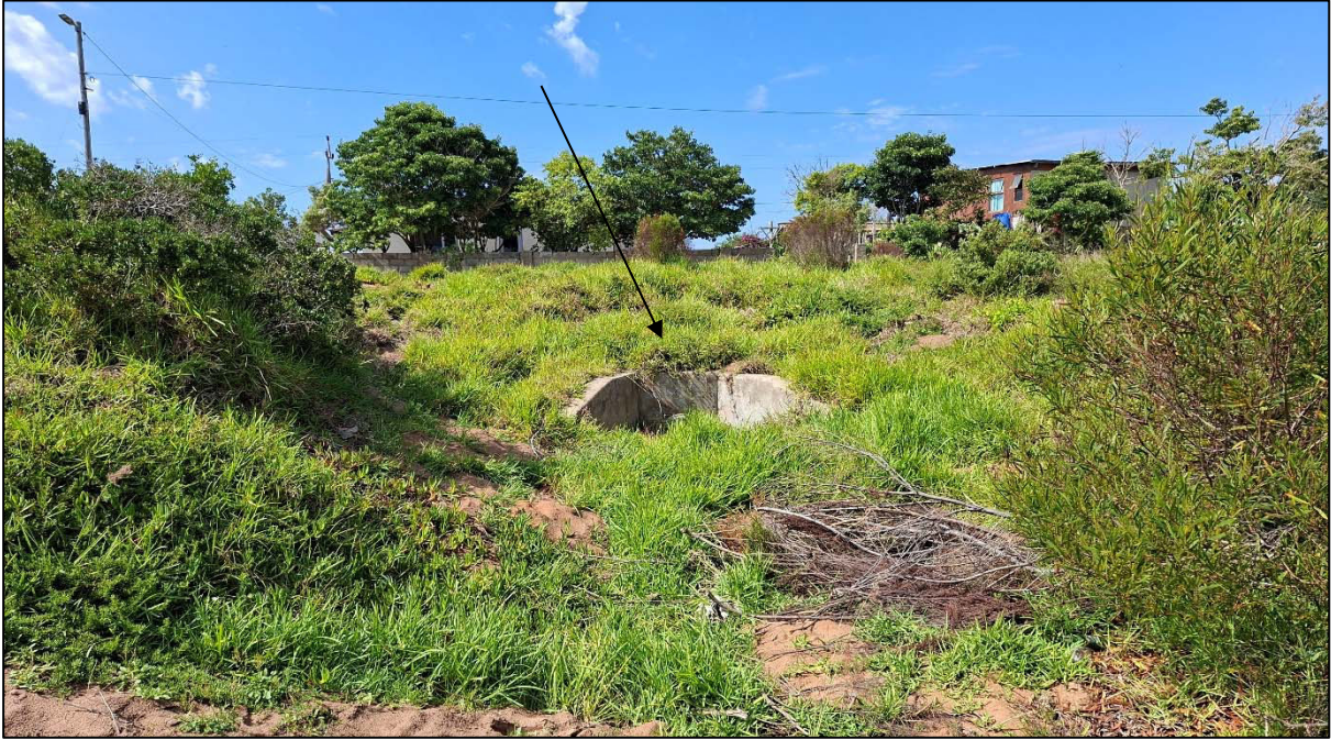
Figure 11: Stormwater pipe culvert under road on eastern boundary of Erf 2686
