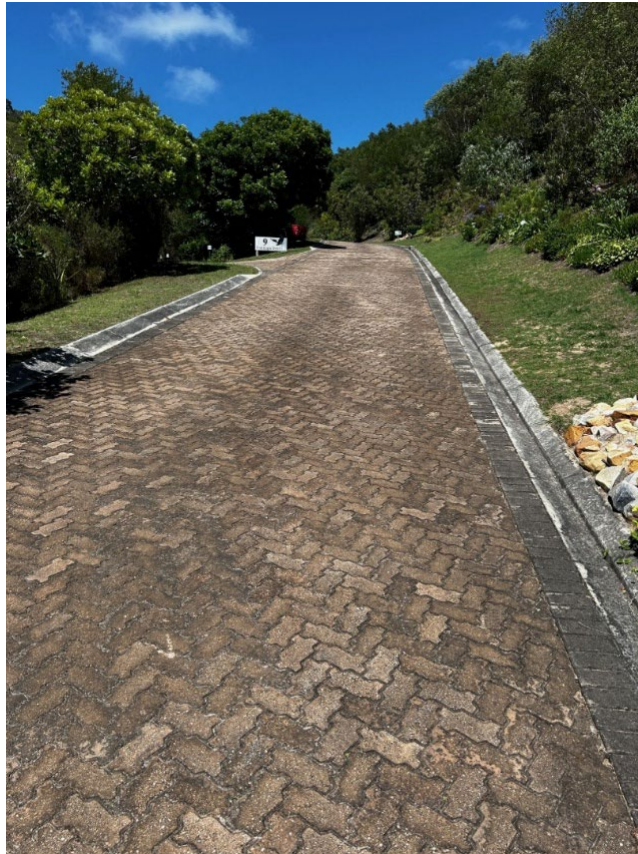
FIGURE 4: TYPICAL MAIN ROADWAY PAVING
