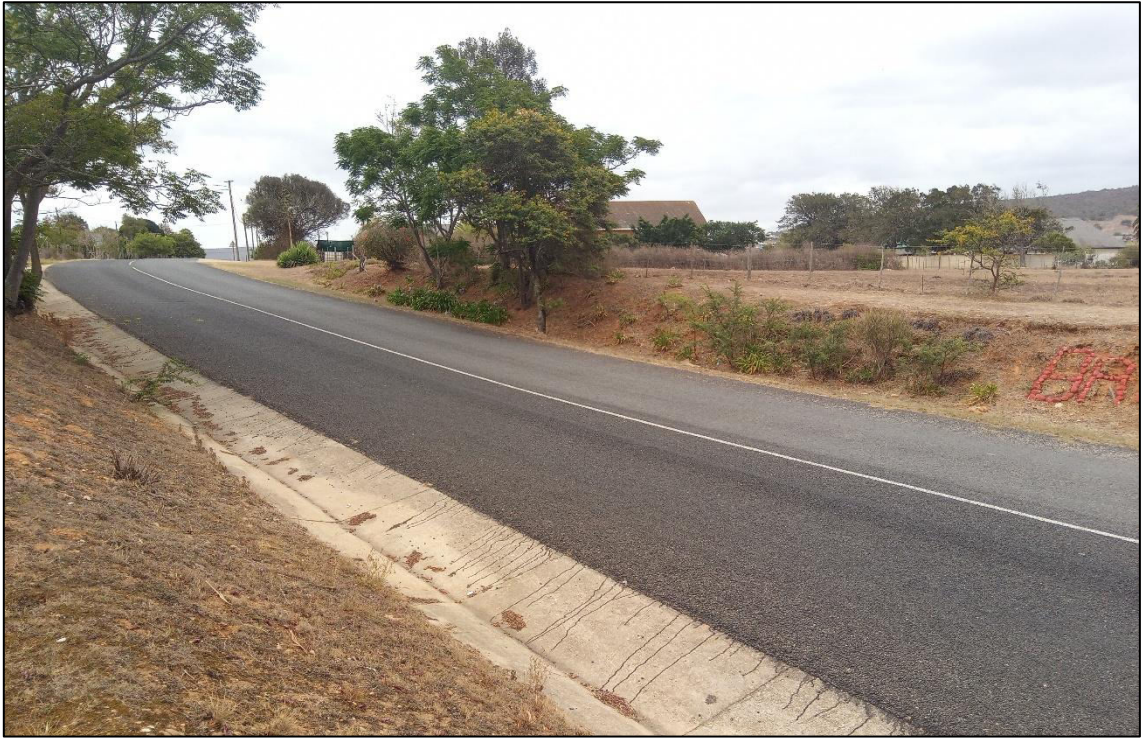
Road leading into Bradwag. The pipeline would be in the road reserve on the far side of the road.
