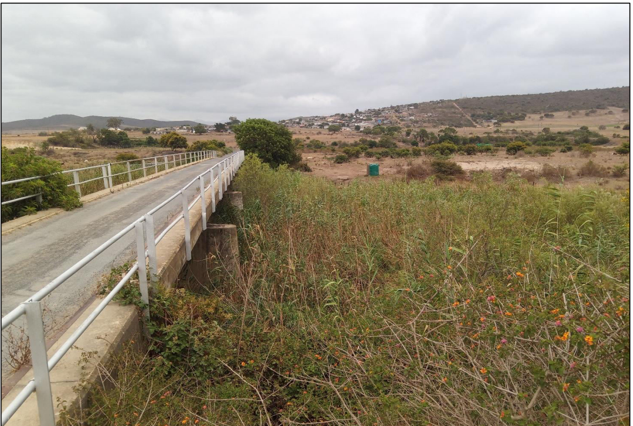
Looking north across the Brandwag River bridge.
