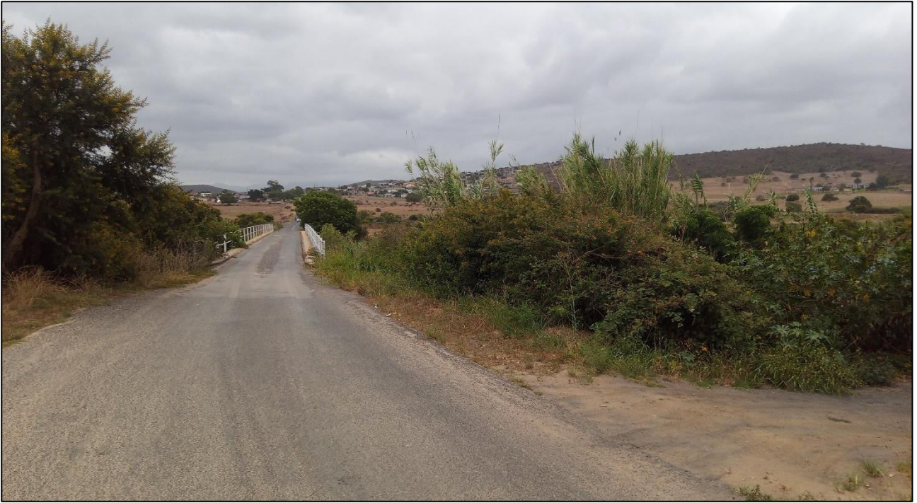
View north across the bridge over the Brandwag River. The pipeline would approach the bridge from the right hand side in this view.
