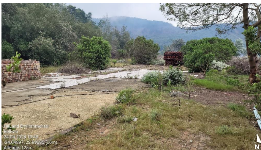
Remaining foundations of burnt home
