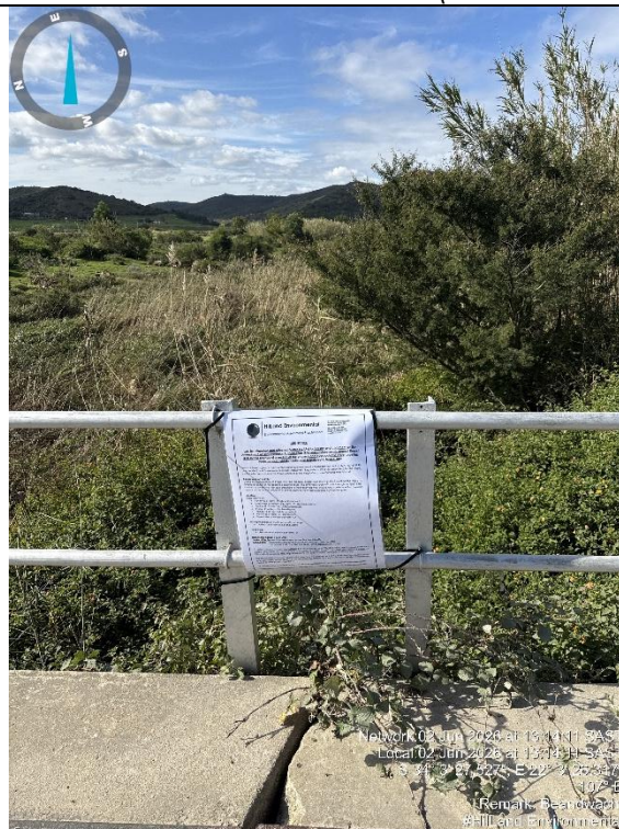
Site Notice on the existing single lane bridge (-34.057552° | 22.057232°)
