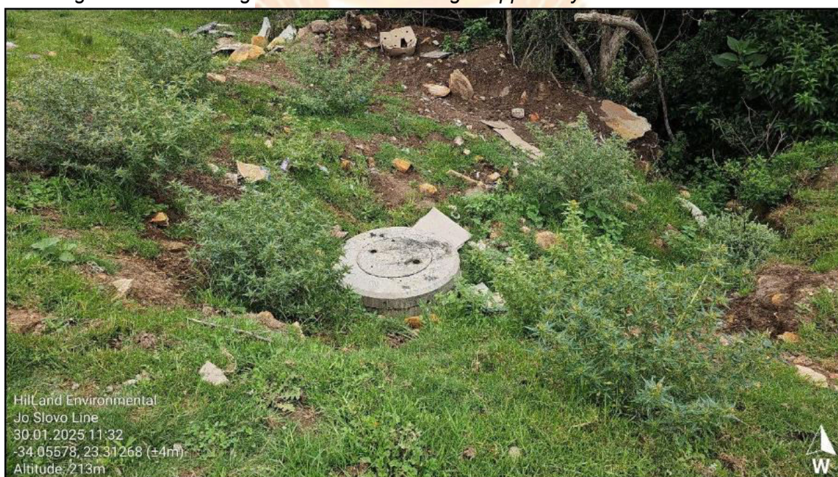
Figure 3: Sections of line have been undercut and eroded which requires repairing.
