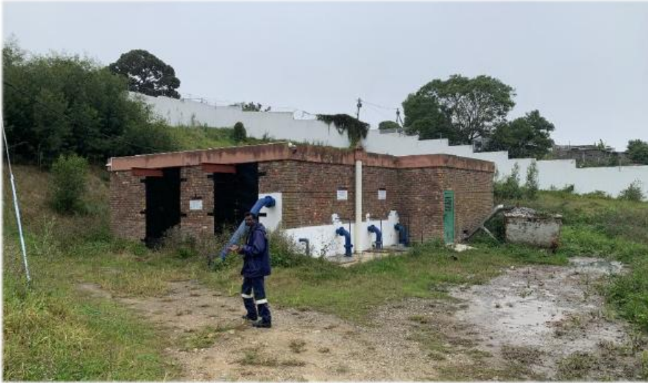
Figure 14 : Overview of Pump Station Site
