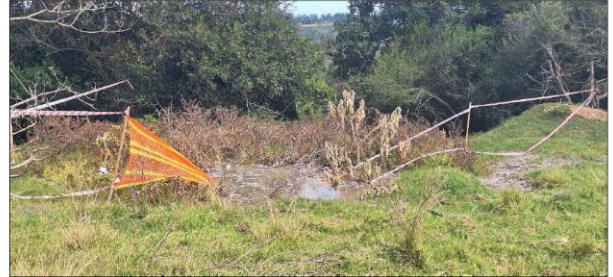
Plate 4: A photograph taken of the overflowing sewer manhole which directly flows into Rip 2.
