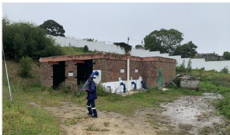
Figure 14 : Overview of Pump Station Site
