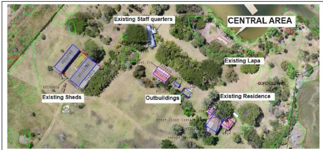
Figure 15: Drone photo showing the existing structures in the central area of the property
