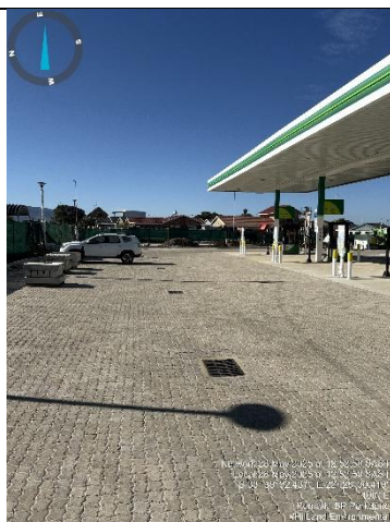
Forecourt paving and stormwater infrastructure installed.
