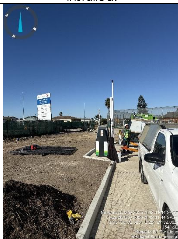
Installation of the fuel pumps in process.
