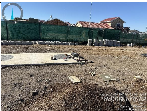
Shaping and rehabilitation started.
