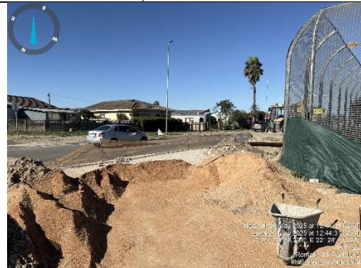
Paving in process at Golf Street entrance.
