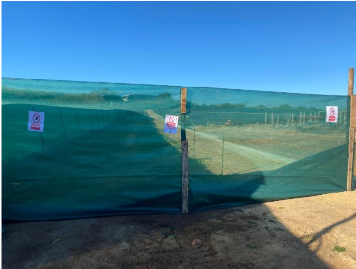
Figure 8 Area above the retaining wall demarcated after discovering that it was outside the property boundary (photo HillLand Environmental).
