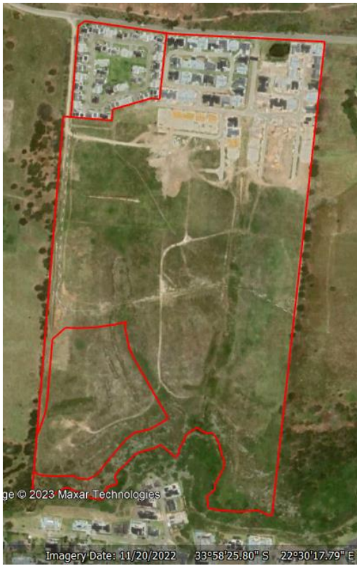
Latest 2022 Google Earth image construction in phase 1 and 2. The remainder of the property consists of some alien invasive vegetation, and cultivation fields that are baled annually.
