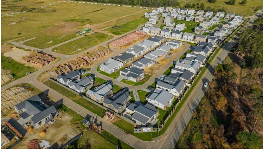
Drone footage over Phase 1 and 2 of Kraaibosch Park (Cape Estates, 2023)
