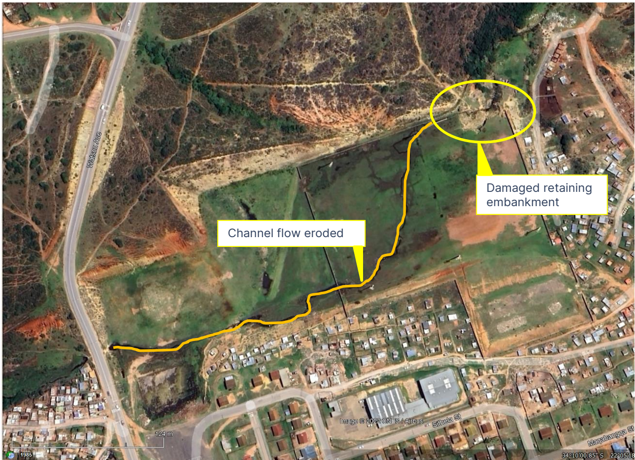
Figure 4-4: Damaged attenuation measures
