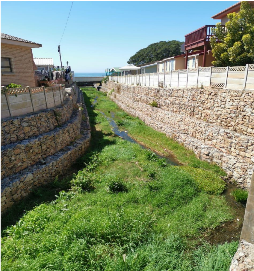
Figure 3-3: Boland Park existing gabion structure
