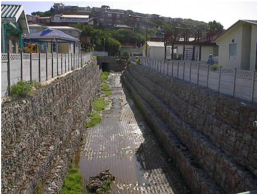
Figure 4-6: Existing Stormwater Channel Profile to be adopted
