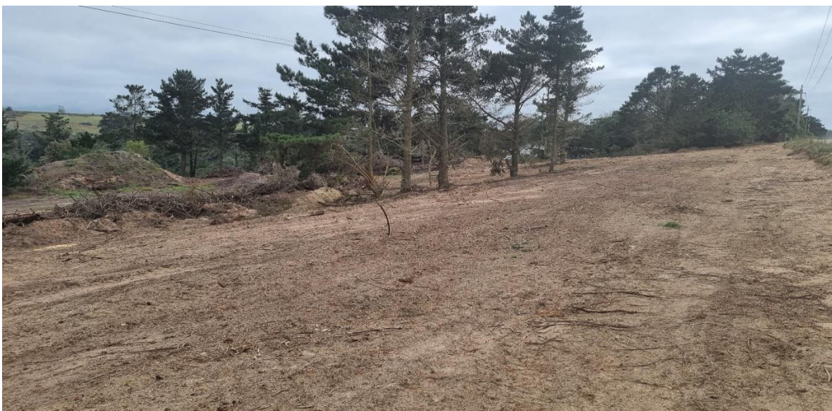
Photo 1: Cleared area at the front section of the property.
