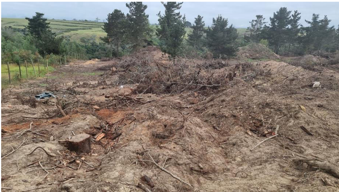
Photo 2: View of the extent of soil disturbance and plant debris indicate that the area was cleared by heavy machinery.
