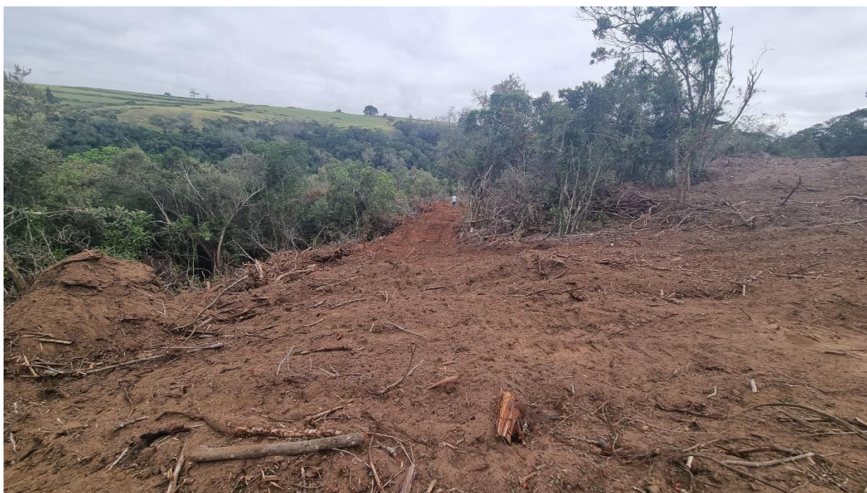
Photo 4: The road that was cleared on the property.
